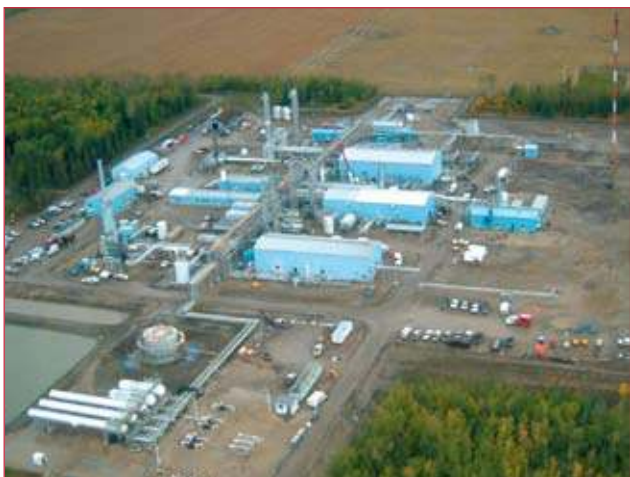
Figure 1. Wembley gas plant.
